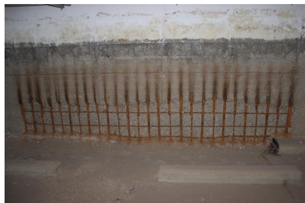
Figure 5. Severe corrosion of reinforcing bars in the retaining wall of the basement.
