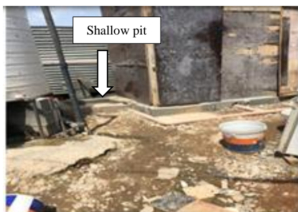
Figure 5. Shallow pit used to accumulate biological waste
