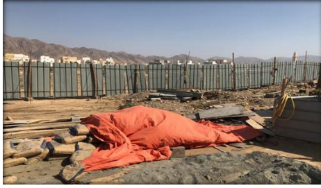
Figure 1. Construction site in Muscat surrounded by a fence
