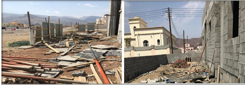
Figure 2. Construction site in Muscat surrounded by a fence
