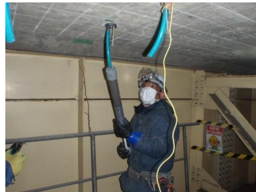
Figure 11. Injection of mortar material
