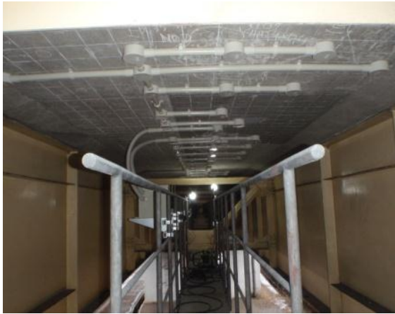
Figure 14. The proposed corrosion mitigation system
