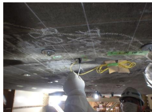
Figure 13. Installation of TW sensor
