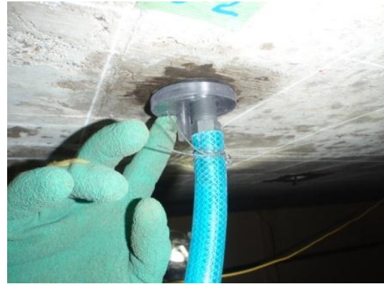
Figure 10. Installation of packing
