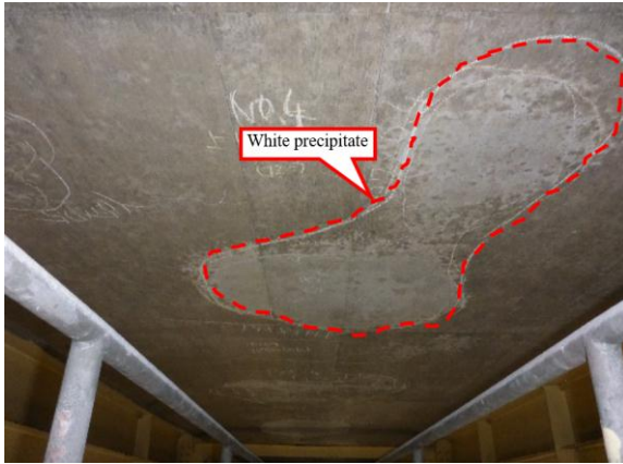
Figure 4. Status of the deck
