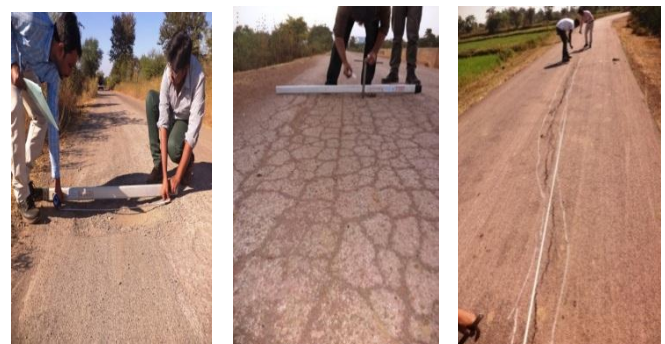
Plate 5: High severity Alligator cracking and rutting
