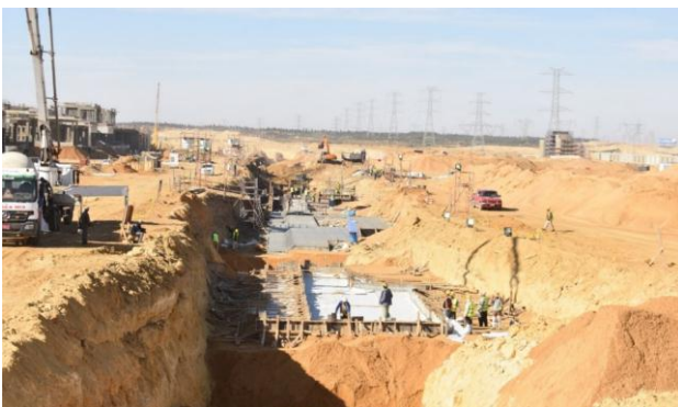
Figure 5. Utility tunnel construction "New capital of Egypt"
