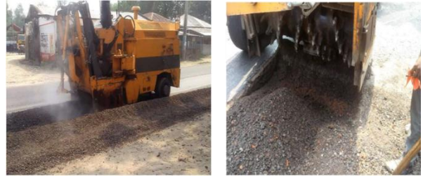
Figure 10. Using of asphalt milling machine.
