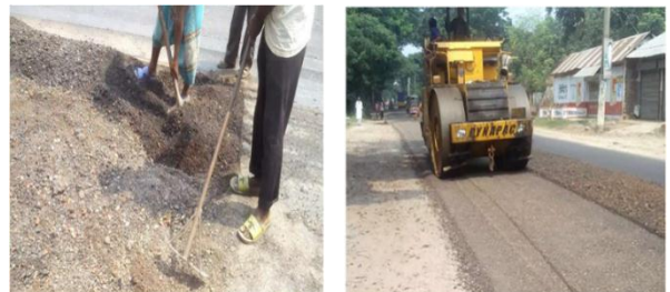
Figure 11. Levelling and compacting road surface
