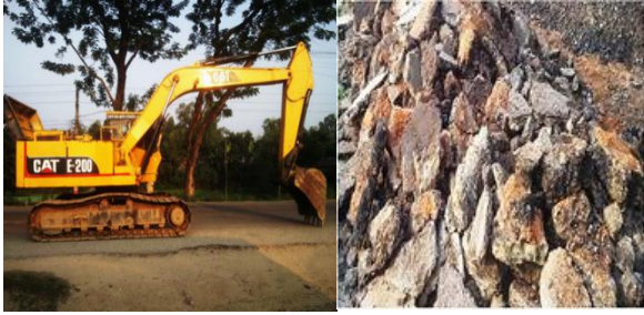
Figure 12. Using of excavator to excavate road surface.
