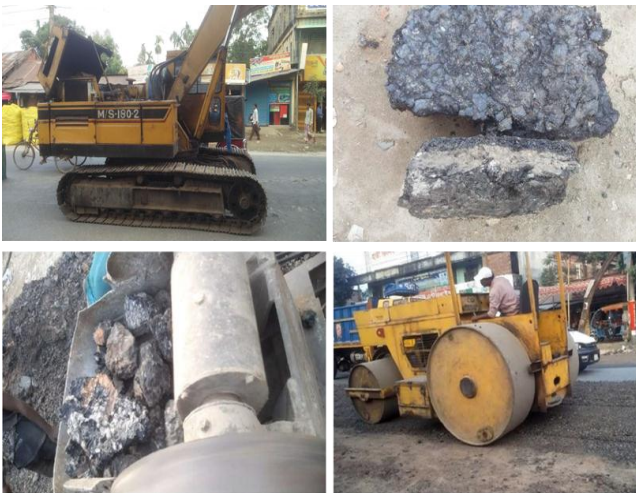
Figure 14. Excavate, crush and re-compact road surface
