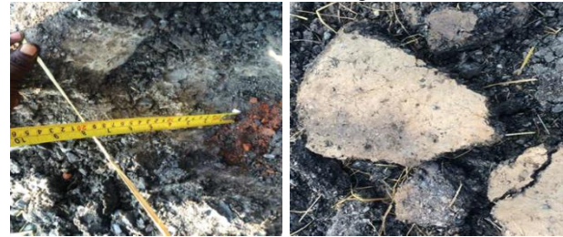
Figure 2. Asphalt Layer Thickness 200mm
