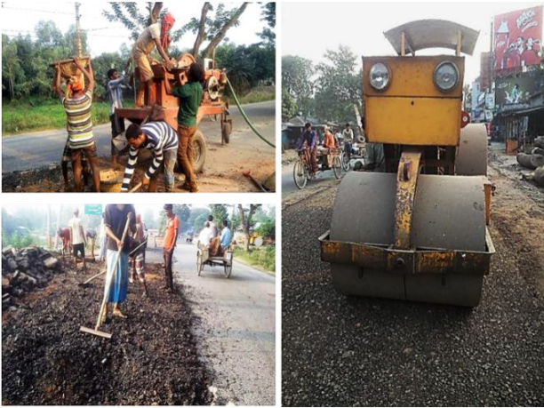
Figure 13. Levelling and compacting road surface
