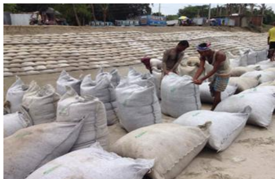
Figure 13. Counting and lengthwise placing of filled geo-bags
