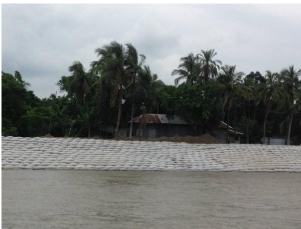
Figure 15. Placing of geo-bag
