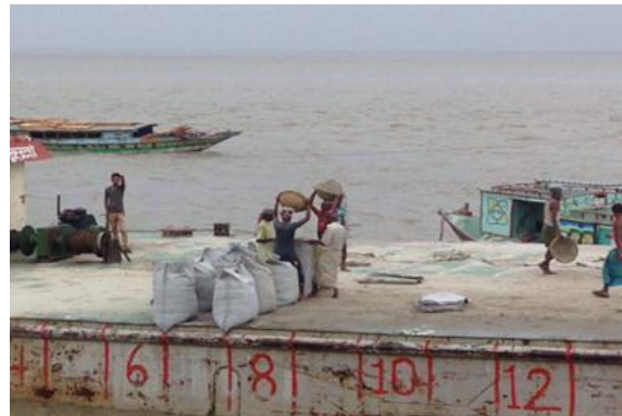
Figure 12. Geo-bags are being placed on the barge according to position
