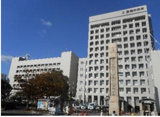
Figure 2. Full view of Toyohashi city hall.
