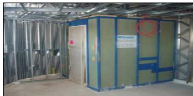
Figure 16. Typical Non-load bearing Module (PODs); courtesy – (Lawson, 2014)
