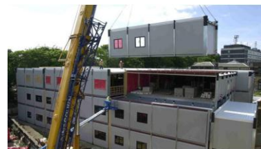
Figure 12. Volumetric (3D) Modular Construction; courtesy - http://www.theconstructioncentre.co.uk
