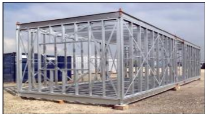
Figure 14. Partially open-sided module; courtesy – (Lawson, 2014)
