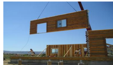
Figure 11. Typical Panelized Modular Construction, courtesy - http://www.grizzlylogbuilders.com
