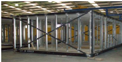
Figure 15. Typical Open-sided Module with corner post, courtesy – (Lawson, 2007)
