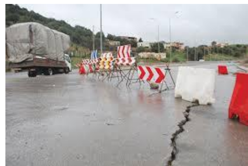
Figure 4. Longitudinal fissure caused by a lack bearing of structure of road by fatigue phenomenon
