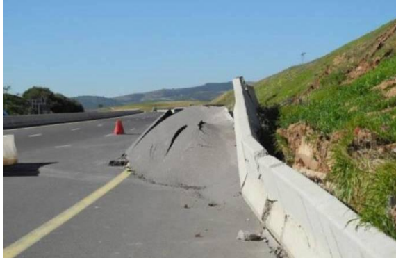
Figure 6. Settlement of bank caused by landslide
