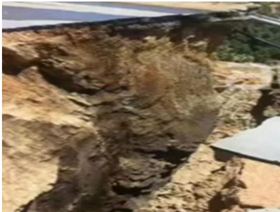
Figure 7. Collapse caused by a geological variation in the soil and water infiltration
