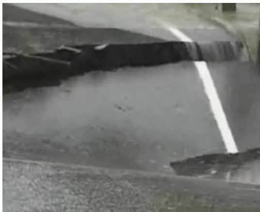
Figure 8. Settlement of soil caused by water infiltration and water saturation of soil (bad drainage)
