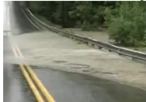
Figure 3. Flooding of road caused by absence of rainwater drainage
