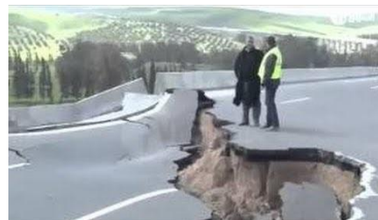
Figure 5. Collapse of road caused by settlement of soil
