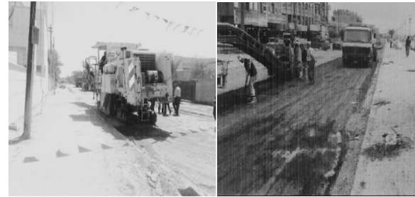
Figure 2: Milling of Asphalt Pavement of Roads in Baghdad
