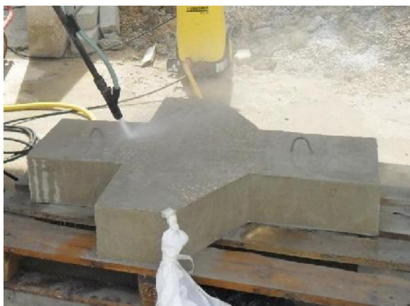
Figure 1: Surface Treatment by Sandblasting
