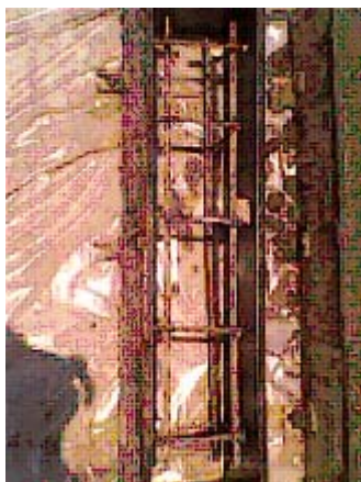
Figure 7: Beams Before casting
