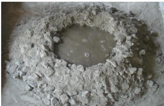
Figure 1: Mixing of Concrete
