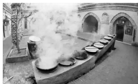
Figure 4. Crossing the mountain stove. It consists of a row of stoves connected in series with 7-8 stove eyes. The firewood is burned at one end of the stove and the heat passes through the hearth to each stove.
