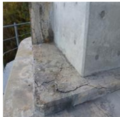
Figure 3. Concrete Jacketing
