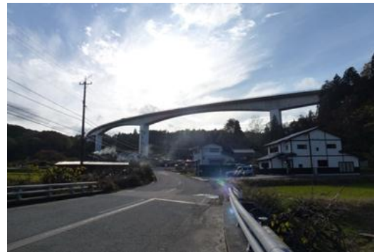
Figure 2. Overview of objective bridge
