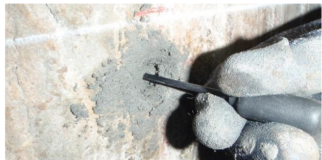
Figure 10. Wire sensor after installation
