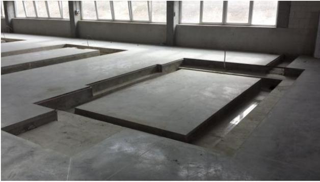
Figure 1. Foundation for an industrial machine [source: sigma-projekt.pl]
