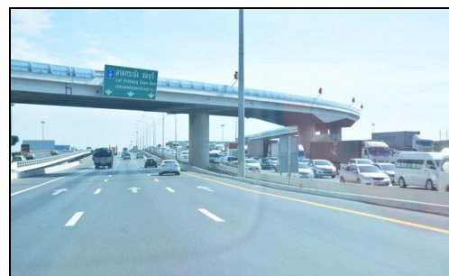
Figure 5. Problems on roadside hazards: height of concrete barrier
