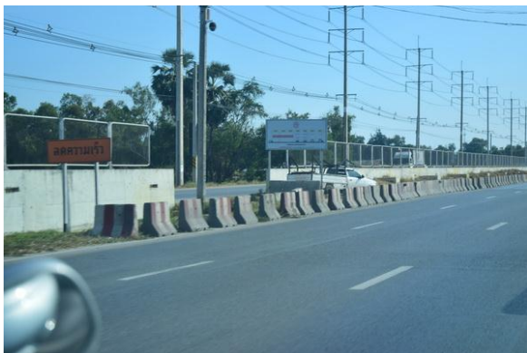
Figure 8. Other problems: roadside activities and hazard.
