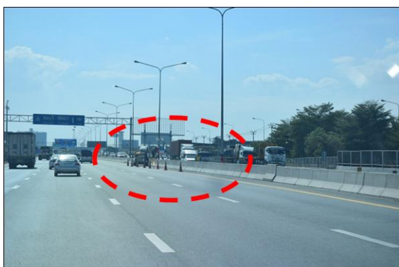
Figure 9. Other problems: roadside activities and hazard.
