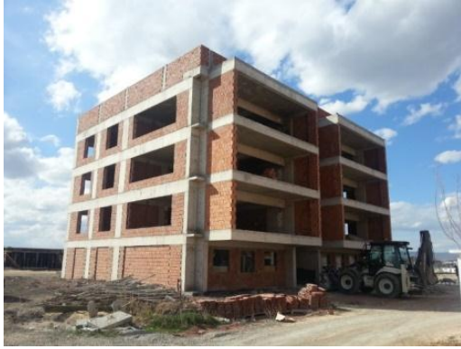
Figure 1. General view of the building
