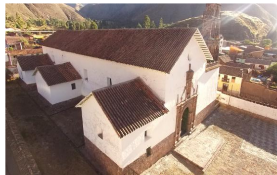
Figure 8. General view of the church.
