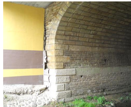
Figure 2. Damaged bridge portal.
