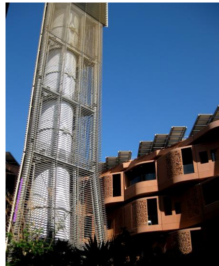
Figure 5. Masdar wind tower and residences with screens and photovoltaic panels.
