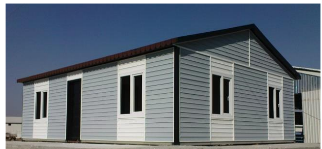
Figure 1. Photo of prefabricated housing
