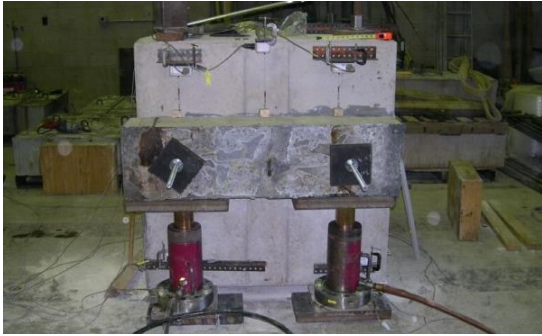
Figure 6. Assembled precast paving notch system (Phase 2).
