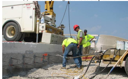
(b) Anchoring stainless bars to the abutment
