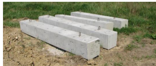
(a) Precast paving notches before placement
