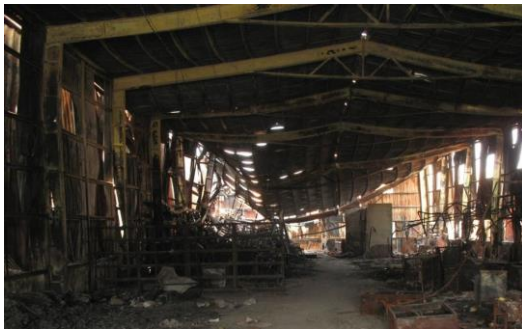
Figure 1. Mountain-shaped structural system of metal houses.
