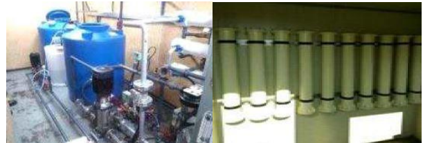
Figure 4. Current situation of construction for water treatment integrated management system.
