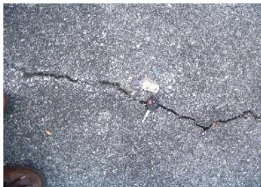
Figure 10: Ideal Time for Crack Filling
