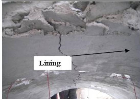
**Figure 18: Cracking In The Mortar Joints at the Level Of The Spandrels On The Extrados**
