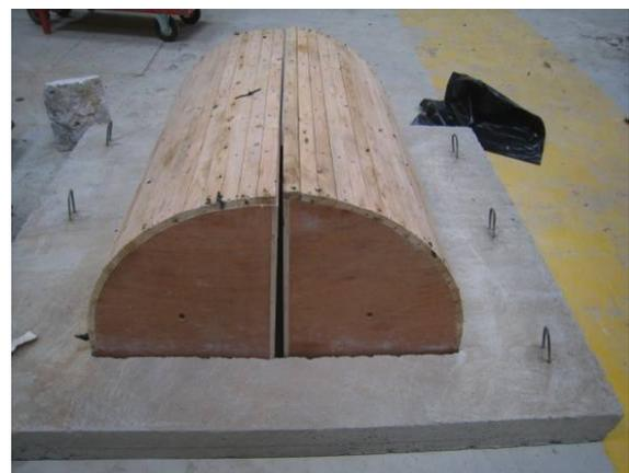
of two juxtaposed parts, with each corresponding to a half-vault. This arrangement facilitated the removal of the formwork after construction was completed. Millstone blocks of various shapes were arranged on the arches to create a mesh. The blocks were cut and trimmed by stonecutting specialists. The vaults were subsequently hand-built, as shown in Figure 12.
