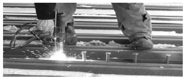
Figure 1: Shear Connectors
