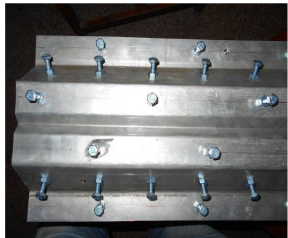
Figure 3: Deck with Bolts
