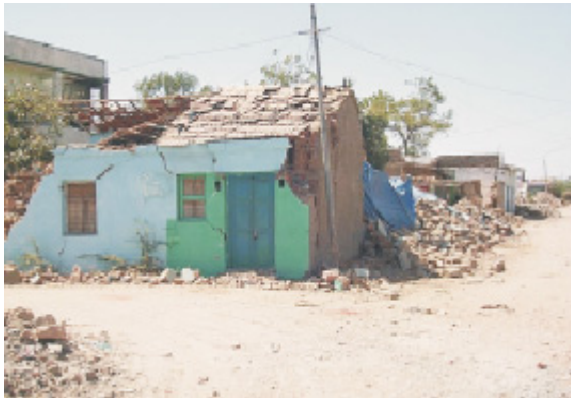
Figure 1: Stone Masonry with Tile Roof
