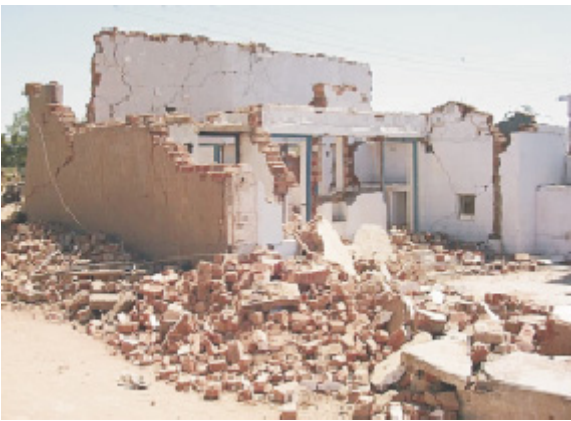
Figure 2: Heavy Stone Masonry Walls That Had No Reinforcement
