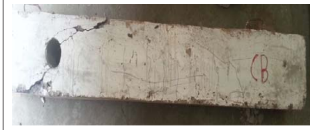
Figure 22: Cracking Pattern for Control Beam
