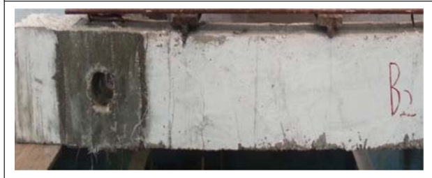
Figure 24: Cracking Pattern for Beam 2
