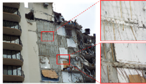
Fig. 11. Wind-resistant wall of western section left at accident site.
