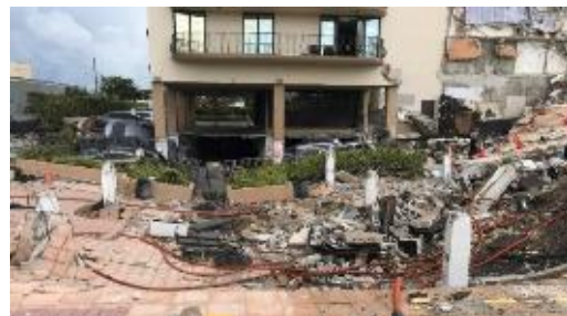
Fig. 11. Wind-resistant wall of western section left at accident site.
