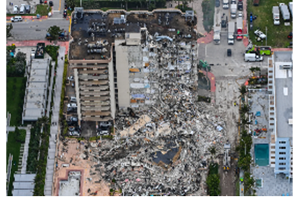
Fig. 3. Collapsed site of the Champlain Towers South.
