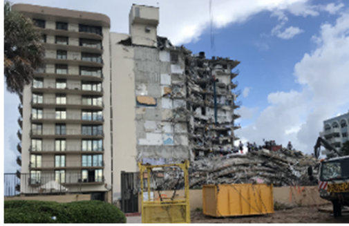
Fig. 8. Western section remaining after the accident.
