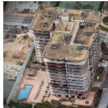
Fig. 1. Champlain Towers South Condominium.
