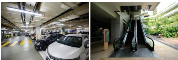
Figure 14. KTPH Sensors in parking and stairs.
