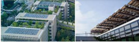
Figure 13. KTPH Solar panels installed.
