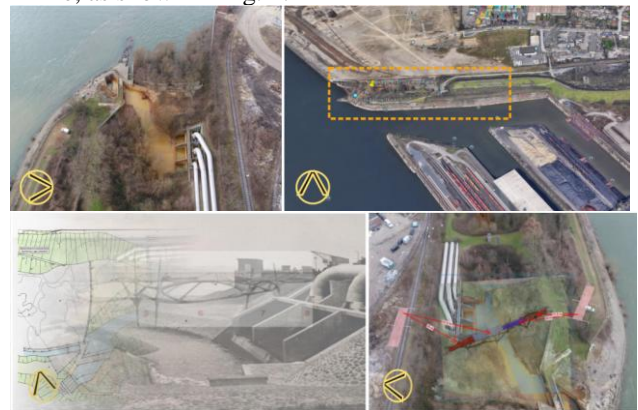
Figure 1. Site view of the park (left), digital twin for the bridge (middle), and assembly location. Source: ©Thomas Spiegelhalter.
